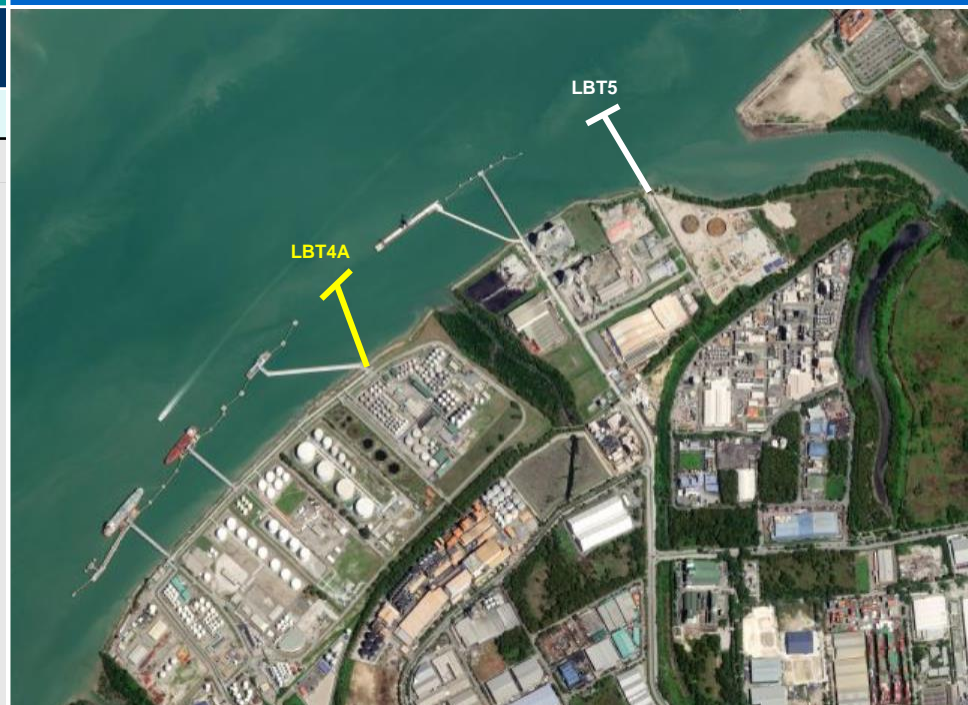
To commence construction of Liquid Bulk Terminal 4A (LBT 4A) in 4Q22
