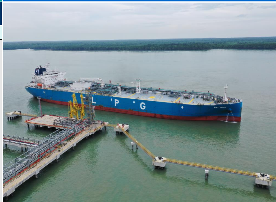
First Very Large Gas Carrier (VLGC) to berth at newly completed Liquid Bulk Terminal 5 (LBT5)
