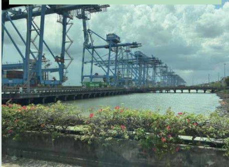
Current condition near B16 @CT
