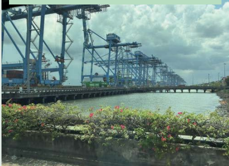
Current condition near B16 @CT
